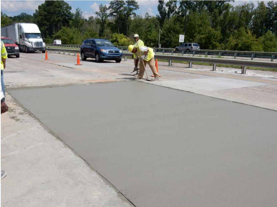
**Figure 2 Second Field Trial of EdenCrete™ being undertaken on the I-20**
