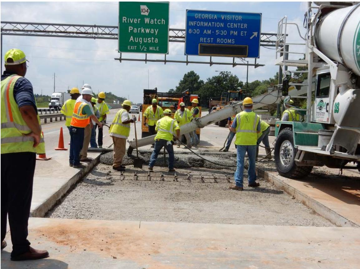
**Figure 1 Second Field Trial of EdenCrete™ being undertaken on the I-20**
