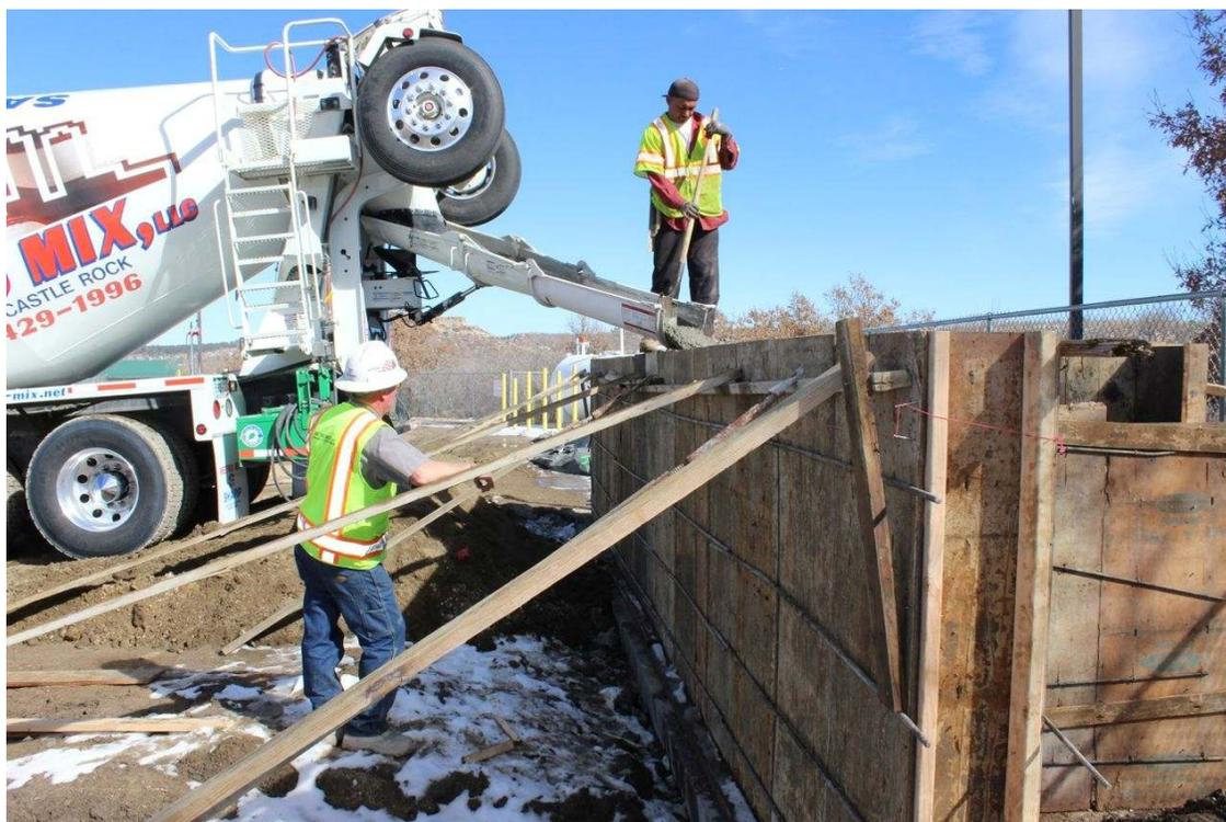
**Figure 4 New aggregate bins being constructed with EdenCrete<sub>500</sub>™**
