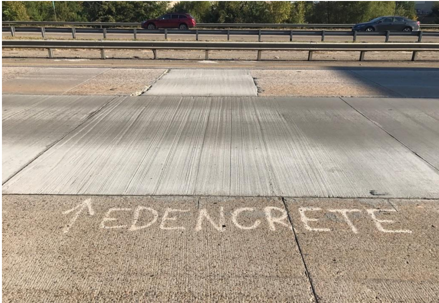
EdenCrete™ – No Visible Cracking
