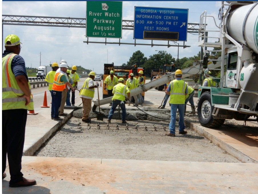
Picture from August 2015 GDOT I-20 Field Test
