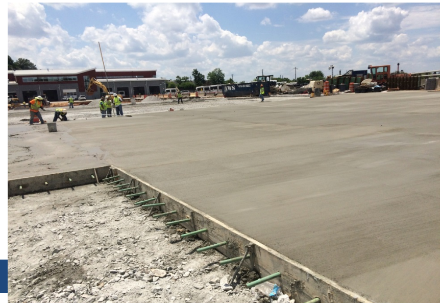
EdenCrete™ Trial Slab
