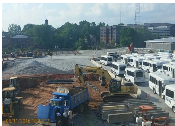
Figure 10. Brady Mobility Facility
