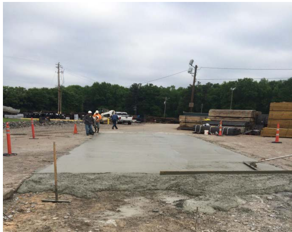
Figure 6. Partially poured first slab
