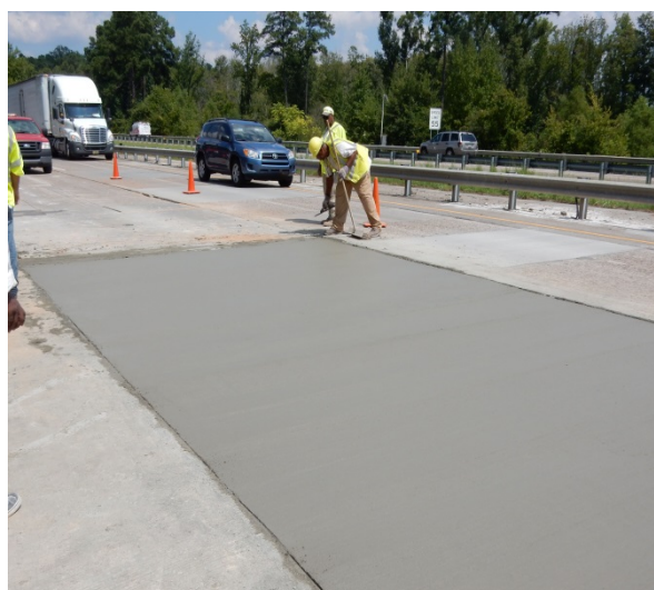
Figure 2 2 nd Field Trial of EdenCrete™ On I-20
