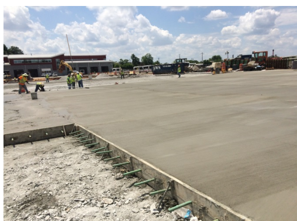
Figure 11. EdenCrete™ enriched slab being installed
