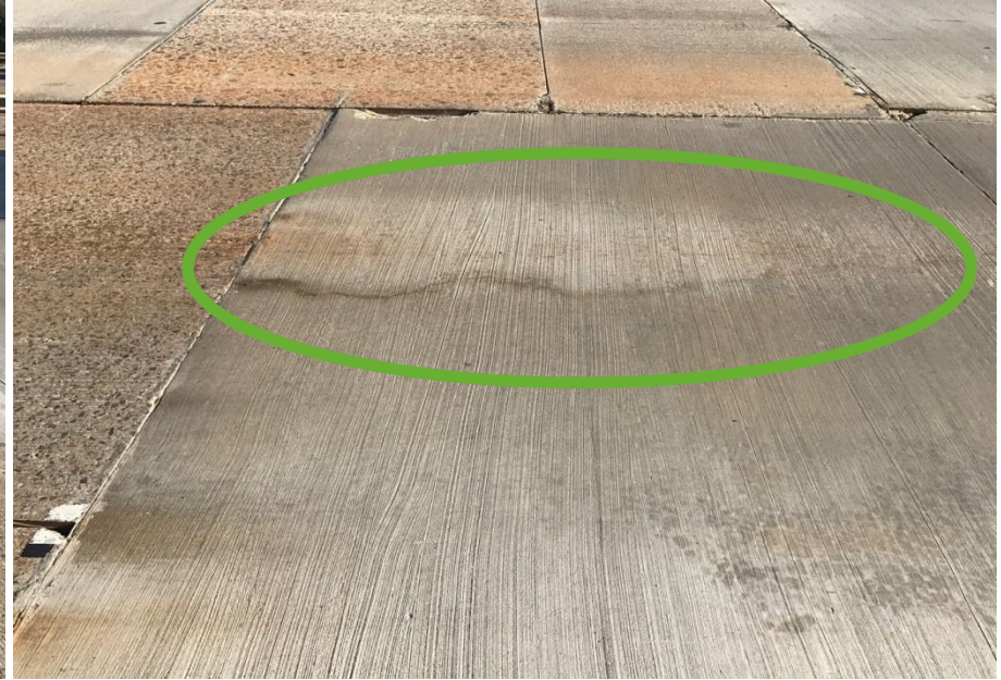
Control – Visible Crack Across Slab
