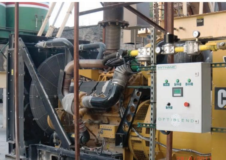
*In order to achieve the maximum reduction in diesel fuel usage, and to maintain the safety and durability of the engine, constant control of the gas is necessary. OptiBlend helps achieve this.*
